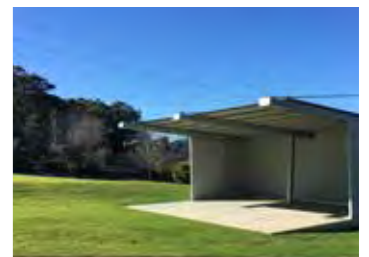
Steel Shelter/Stage on Concrete Slab in turf area
