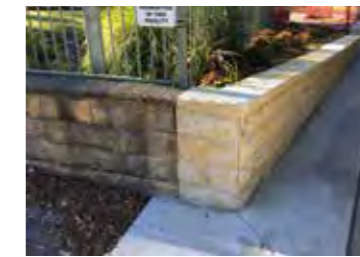
Sandstone capped retaining wall
