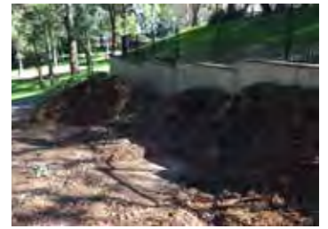
Concrete block retaining wall
