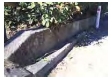
Sandstone block retaining wall
