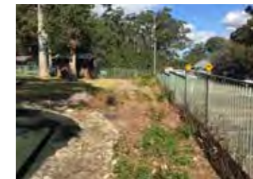
Informal drainage line with rock finish
